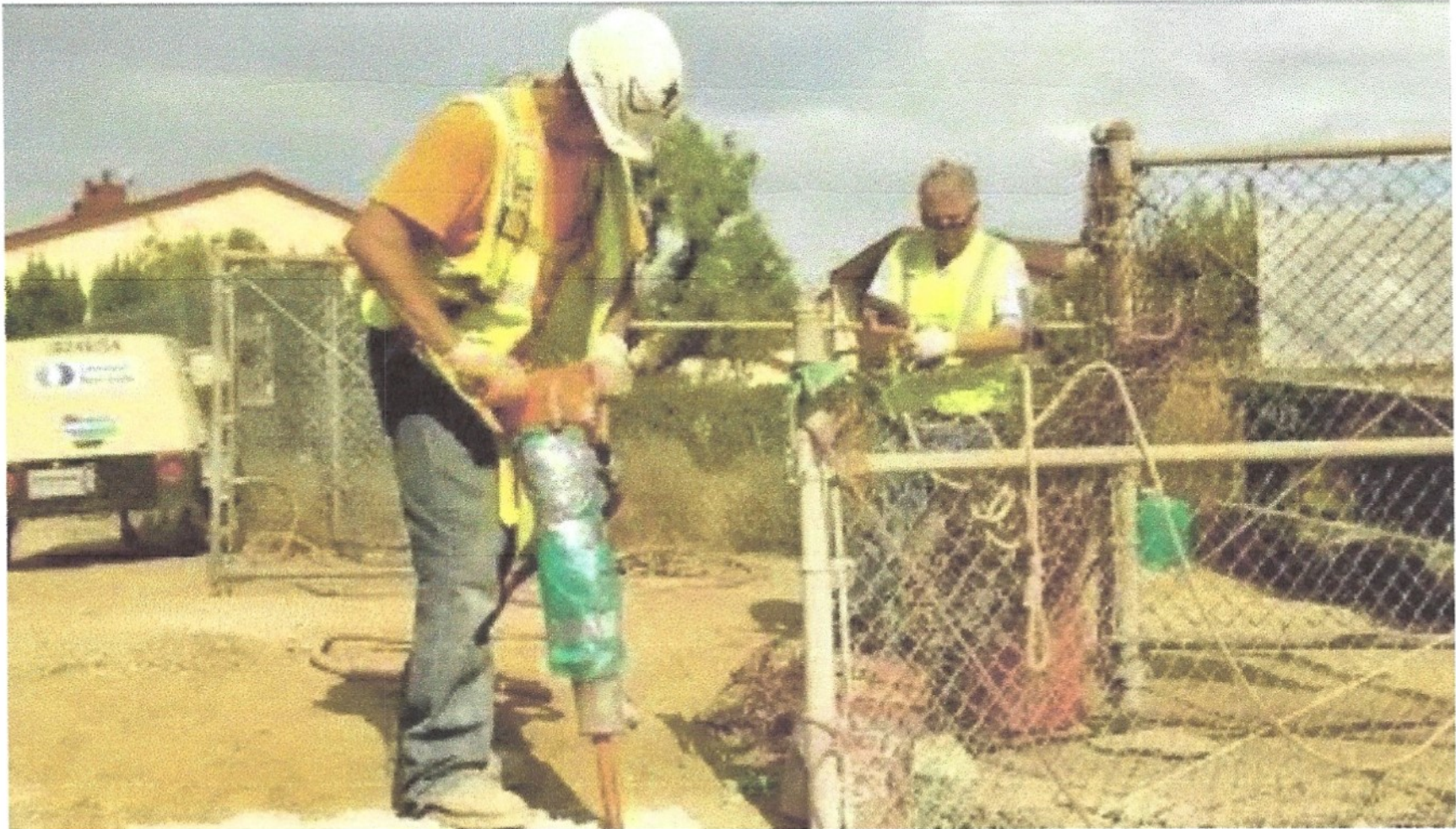
Public works projects come in a wide variety of sizes. (CDABP)
